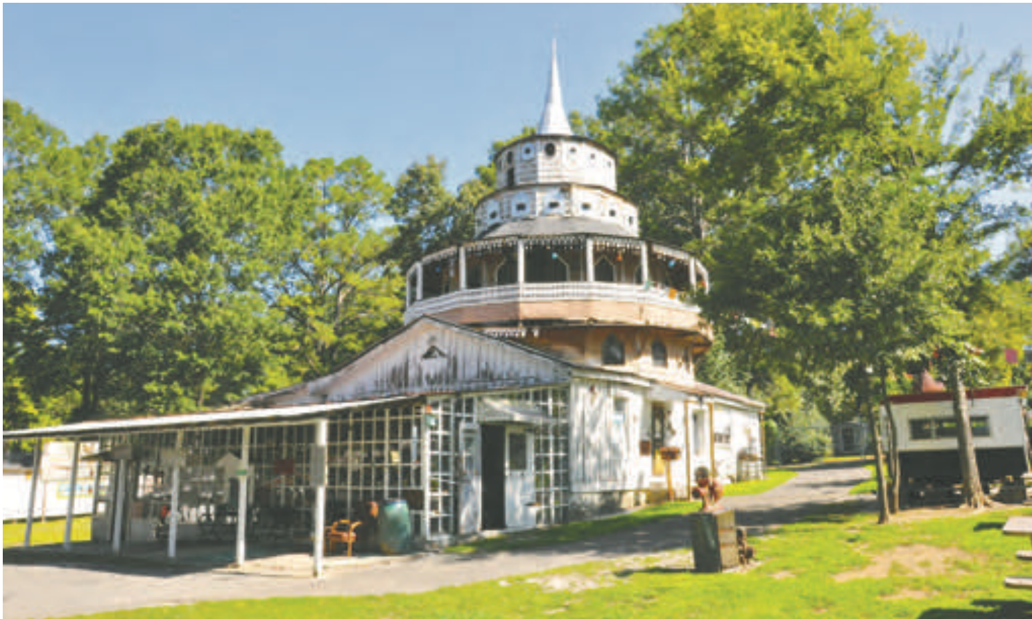
Howard Finster's World's Folk Art Church towers 40 feet and has an odd construction of four floors, 16 sides and a circular staircase — a plan the artist said came in a vision. Built as a place to “preach through my art,” the Paradise Garden Foundation is seeking funds to revitalize the unique building into “iconic conference space.”
