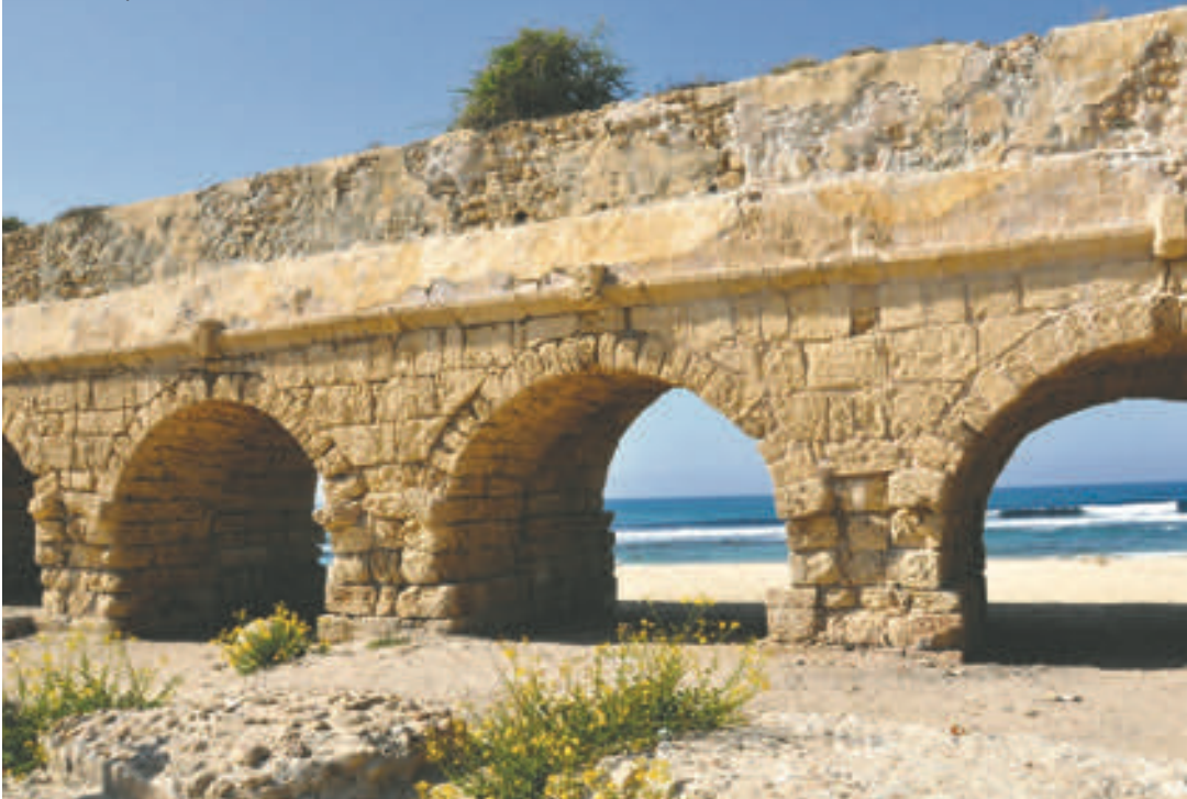
Ancient aqueduct at Caesarea Maritima
